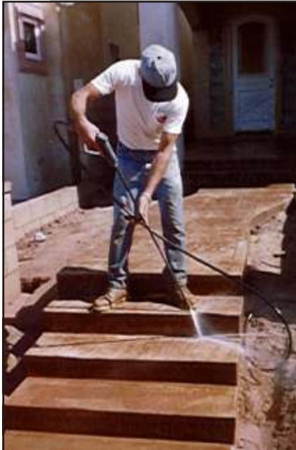
**Clean-up and sealing** the initial clean-up should be done the day you pour, clean all the adjacent areas with water and a scrub brush . Three to five days after installing the textured concrete it must be pressure washed with a minimum 2000 PSI pressure washer. After pressure washing, do any necessary touch-up or chip repair and seal with an acrylic exterior concrete sealer.
