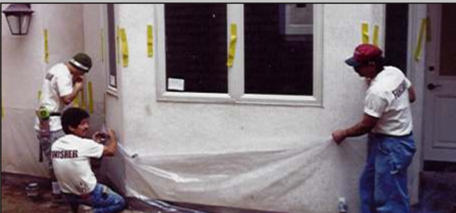
**Obstacles or any adjacent walls and flat work** must be protected from concrete, color and colored release with a clear 2 mil visqueen.
